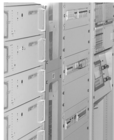
Fig.6. Modular construction of level crossing system type RASP-4
