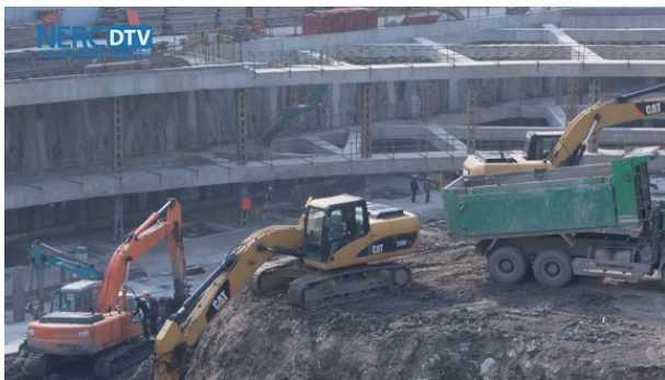
(c) Construction Field.
